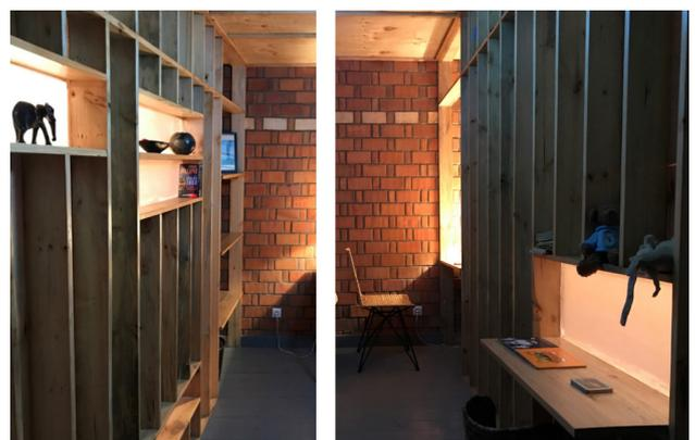
Figure 5 : Interior kids bedroom with both timber slab and timber partition wall
