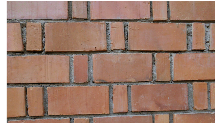
RLB wall before pointing. RLB wall pointing works
